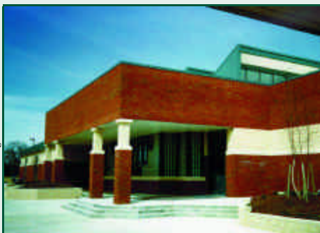
Roof monitors at Clayton Middle School, Clayton, NC.
