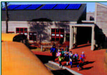
Grid-connected photovoltaic system on Nantucket Elementary School
