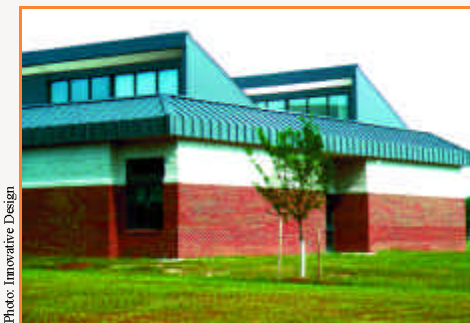
Roof monitor at Clayton Middle School, Clayton, NC
