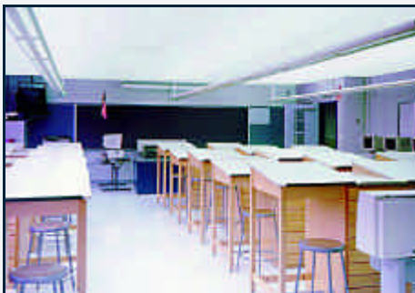
Indirect lighting fixtures
