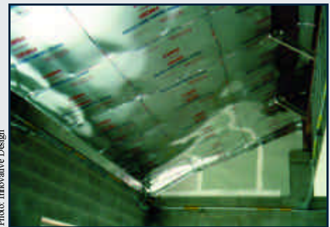
Radiant barrier in roof assembly
