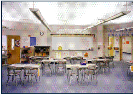
Indirect lighting fixtures
