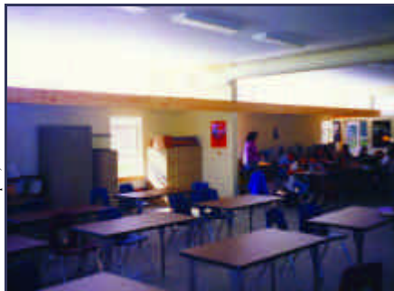
Sun rays bouncing on interior lightshelves onto ceiling
