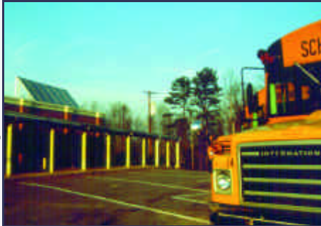
Solar system save energy and helps out environment
